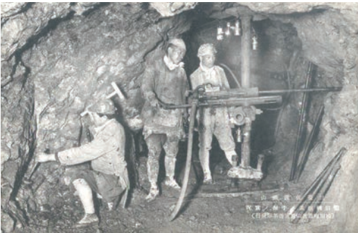
Mining by rock drill and hand at Sado Mine (1930s)
