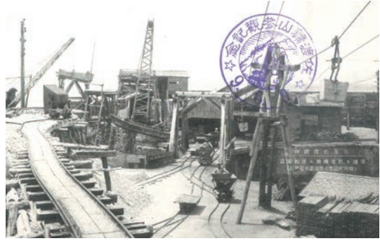
Loading pier before the construction of Oma Port: mine cars and aerial cables used for transportation (circa mid-1930s)
